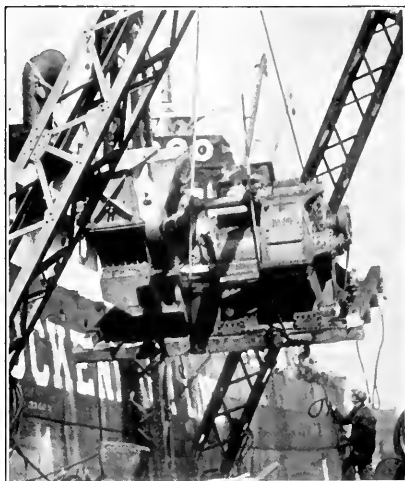
Bauer-Wach exhaust turbine unit being hoisted aboard the steamship Lena S. Luckenbach .
